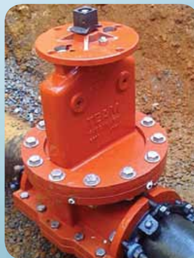
An InsertValve with position indicator plate. Valve can be fitted with gear or handwheel operators.
