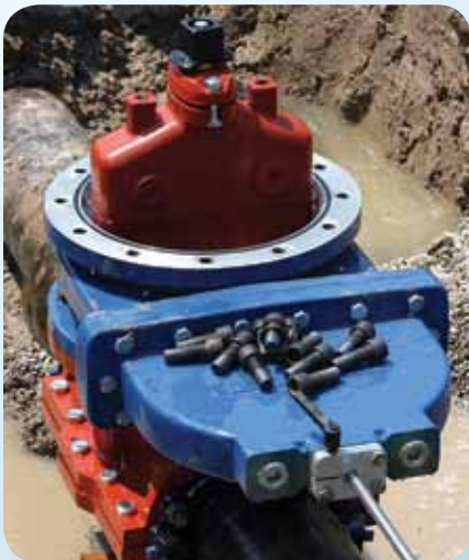
Low-profile bonnet used as line stop.
