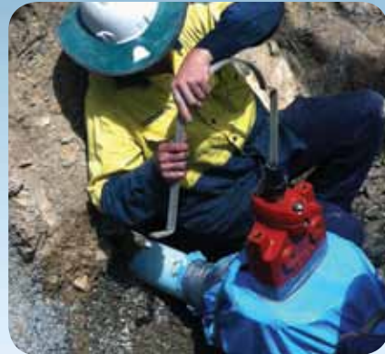
An InsertValve installation under full line pressure.
