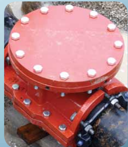
Blind flange installed.
